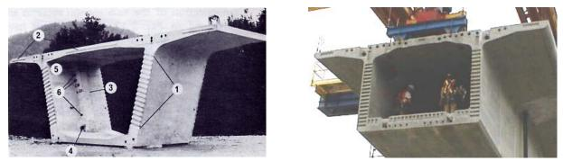
Figure 1 Precast segmental box girder sections. Left: pre-1975 (PTI 1978). Right: 2000
